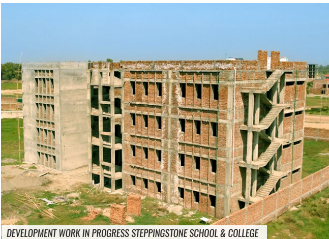
DEVELOPMENT WORK IN PROGRESS STEPPINGSTONE SCHOOL & COLLEGE
