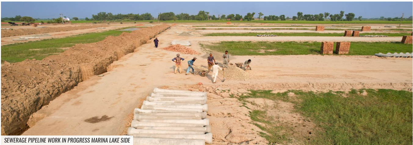
SEWERAGE PIPELINE WORK IN PROGRESS MARINA LAKE SIDE
