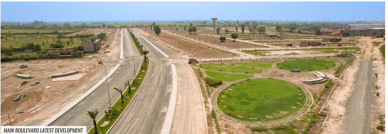
ENTRANCE GATE LATEST DEVELOPMENT
