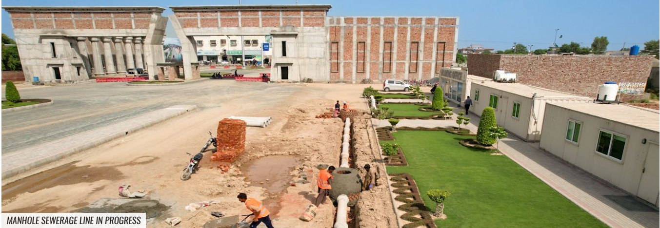
MANHOLE SEWERAGE LINE IN PROGRESS
