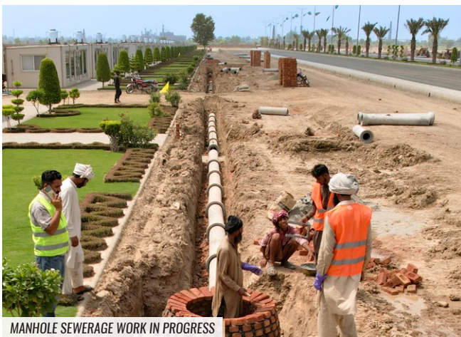
MANHOLE SEWERAGE WORK IN PROGRESS
