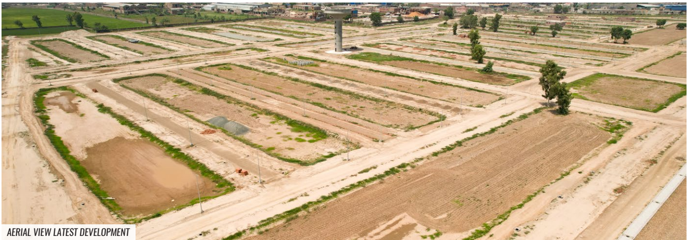
AERIAL VIEW LATEST DEVELOPMENT
