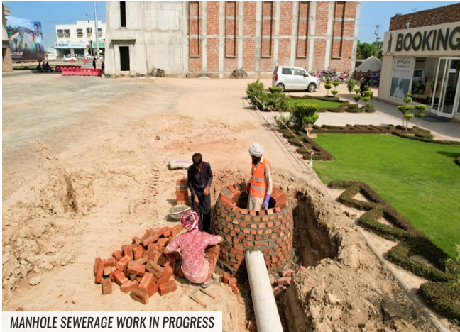
MANHOLE SEWERAGE WORK IN PROGRESS
