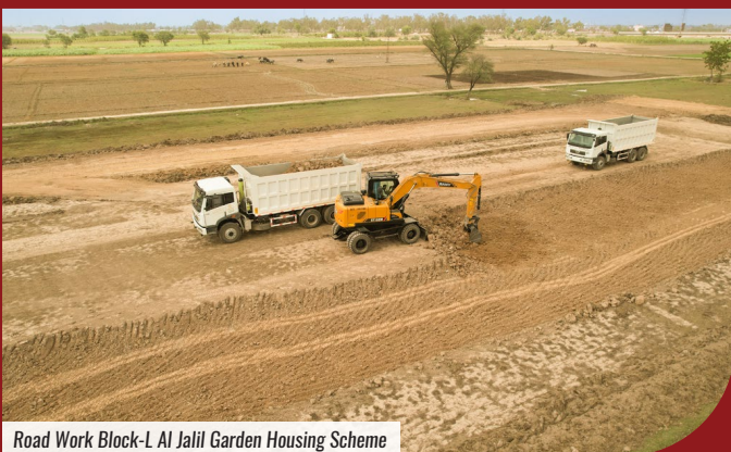
Development Work Aerial View Block-L Al Jalil Garden Housing Scheme
