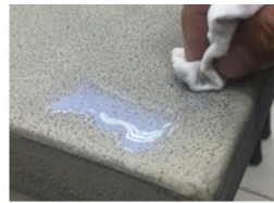
Distribute the DuralCrete protection equally on the surface, using a soft cloth.
