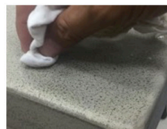
Distribute the DuralCrete protection equally on the surface, using a soft cloth.
