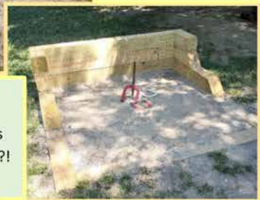
Old and tired original timbers needed to be replaced.
