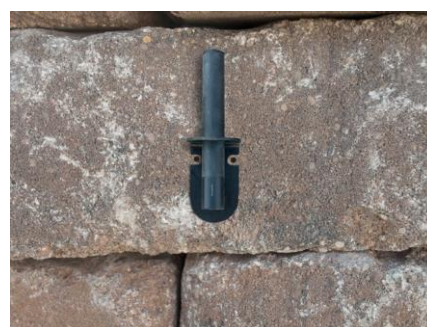
Figure 6.8 – Dry fit the bracket
