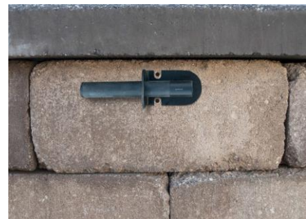
Figure 6.4 – Dry fit the bracket
