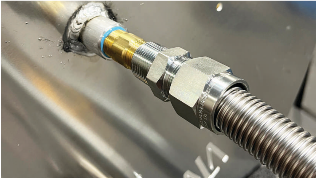
Photo 18: Connecting the Flex Line
