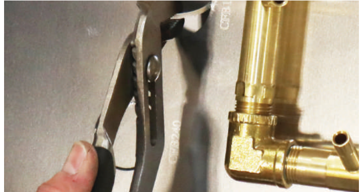
Photo 2: Breaking the Knockouts
