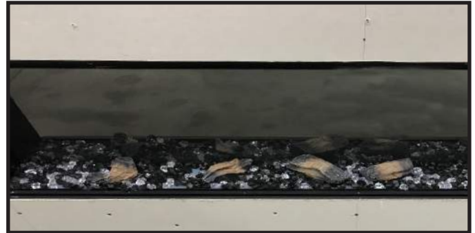
Figure 4.10 Media and Small Logs Installation
