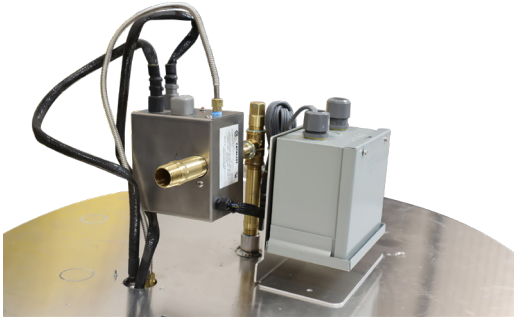
Photo 25: Connecting the 3/4" x 3" nipple to the Platinum Valve
