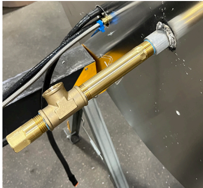
Photo 7: Installing the Drip Leg
