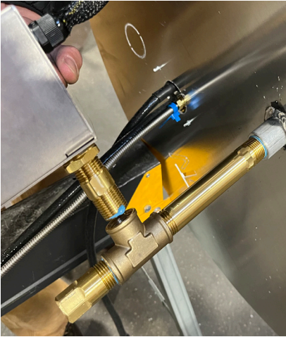
Photo 9: Attaching the Valve Box to the Drip Leg
