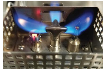
Figure 10.2 – Pilot flame coverage of thermocouple.
