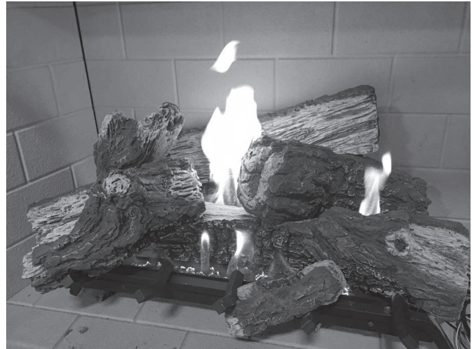
Figure 6.13 - Correct Appearance of Rear Flames
