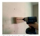
Attach the cleat to the wall useing mechanical fasteners and a type of adhesive. In this example the fireplace specifications and building codes allow for a wood 2 x 4 cleat to be used.
