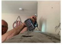
Set the mantel shelf onto the wall cleat and use the screws and screw through the holes into the nailing cleat. Use a machting color patch or grout to fill the holes. Usally the mantel is high enough that no one will see the holes. We recomend not making the holes disapear in case you need to remove the mantel for whatever mason.
