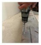
Drill at least 5 holes equally through the top of the mantel at least 1" away from the edge. We recommend starting with a 3/16" masonry bit. Drill all the way through the material.
