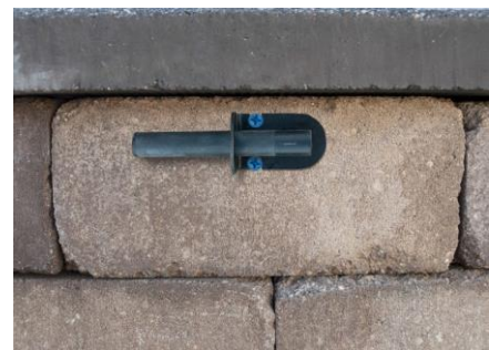
Figure 6.5 – Fasten down the bracket
