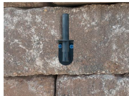
Figure 6.9 – Fasten down the bracket
