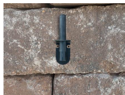
Figure 6.8 – Dry fit the bracket
