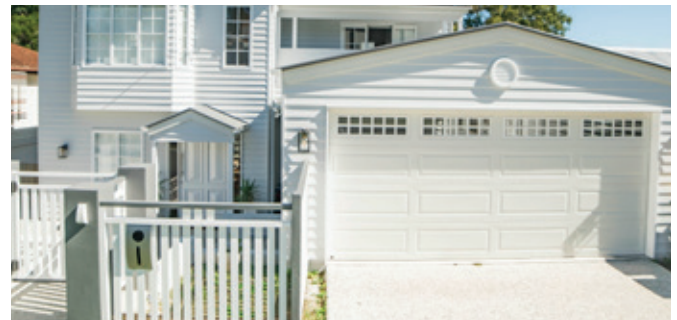
Grange with Stockton windows
