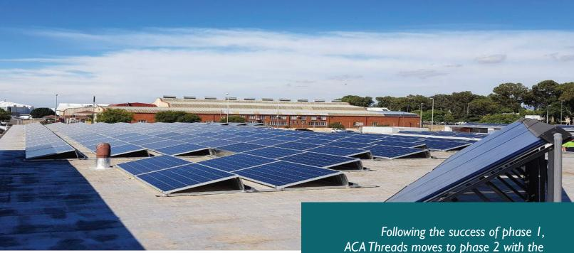
With the rising cost of electricity, and having reaped the benefits of phase I, whereby a I31kWp solar generation system was installed, ACA Threads moves onto phase 2 to further lessen their dependence on municiple power.
