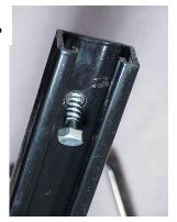
Attach vertical frames to wall using lag bolts. Make sure to attach to studs in wall. Other method of attaching may be needed depending on type of wall. Make sure vertical frames are secure before attaching tier kits
