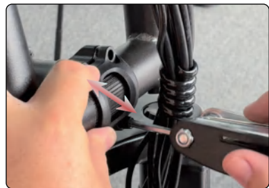
D) First, install the two diagonal screws, and screw them in halfway.
