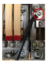
4. Screw down the new cable's shield terminal lug along with the ground jumper lug removed earlier.
