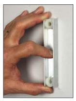
Place bracket channel on wall - Once you have determined the location for the wall mount, use the bracket channel as a template guide to mark the location of the screw holes. (Be sure to place the channel on the wall with the U-shaped spacer on the bottom with the opening facing up. This is critical to allow clearance for the bracket hooks to fully engage the bracket plate).
