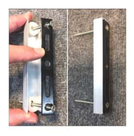
Hold the assembly to the wall and start to thread each screw several turns into the pilot hole before tightening them completely. Drive the screws in almost all the way, then align the plate to the vertical and horizontal centers of the channel. Tighten the screws firmly, **but be careful not to over tighten**. It is best to use a hand screwdriver to do this final tightening.
