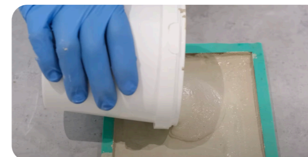
Step Seven Back-fill with AC630/730/830 solid/laminated.
