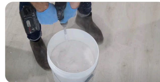
Step Three Mix Together (At the specified 2.5:1 Ratio).
