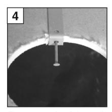
The new fast-fixing clip attached to the speaker covers. This clip attaches the speaker cover to the ceiling.
