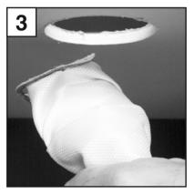
Grasp the cover by its sides and squeeze it inwards to reduce its bulk. Then push it through the aperture with its top uppermost, ensuring that a grip on the fitting clips is maintained throughout the process.
