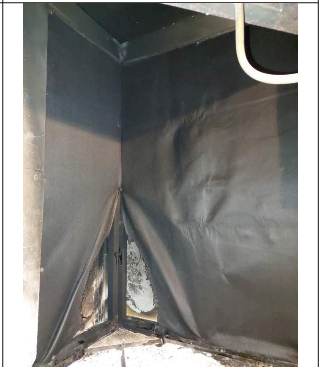
Photograph of the exposed surface after the test
