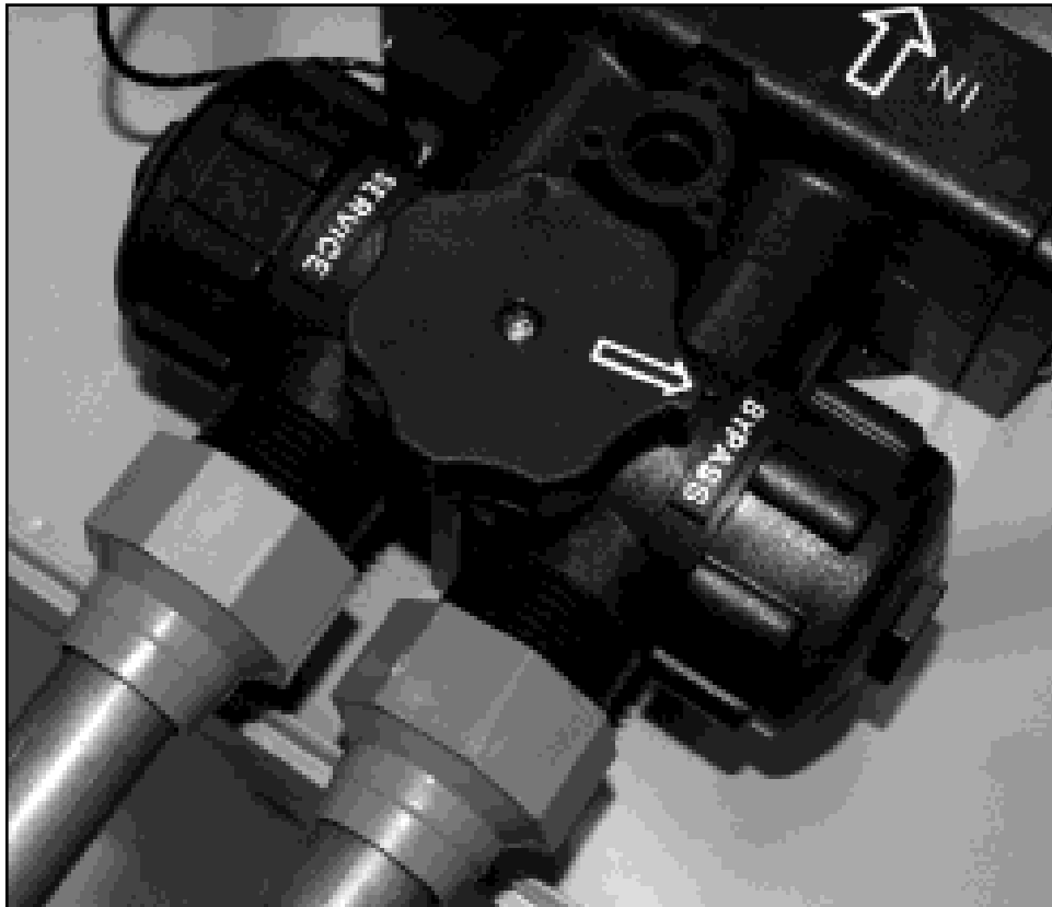
Figure 8: Bypass Valve
