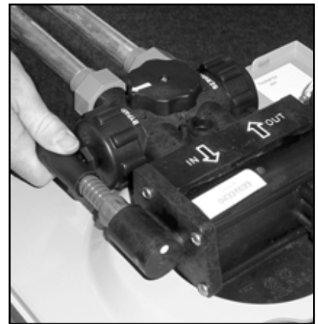
Figure 4: Connect Drain Line
