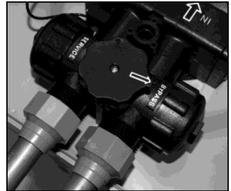
Figure 5: Bypass Position
