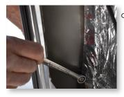
d. Place the Phillips head screw driver over the screw and tighten the nut with the 7/16" socket or wrench.
