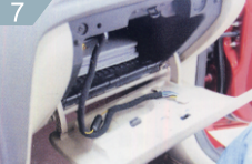
Pull through DSP-1 wiring harness to installation location
