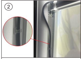
Attach wire clips to the frame. Then route the cable through and secure within the clips.
