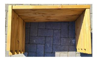
**Step 4:** Now do the same with the final side section, you may need to tap it into place gently before fixing with screws.
