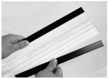
With the longer side on top, fit two the J-channels as far as they can go over the bottom and top edge of the fixture.
