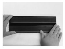
Align the Double ClearVision® piece in between the two J-channel pieces.
