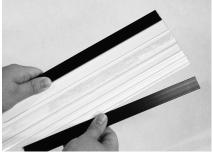
With the longer side on top, fit two the J-channels as far as they can go over the bottom and top edge of the fixture.
