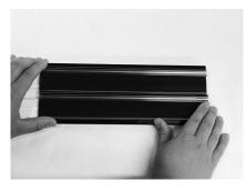
Align the Double ClearGrip™ piece in between the two J-channel pieces.
