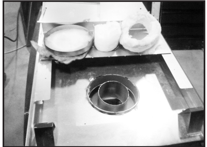
Figure 6.3 Remove and discard the seal cap, insulation donut, insulation plug, and the insulation basket. Attach the first vent section (it will snap into place). Slide the vent gasket onto the vent section and then, up against the appliance. Secure the vent gasket to the appliance with two self-tapping screws found in the manual bag. Note: The vent gasket can found in the manual bag.
