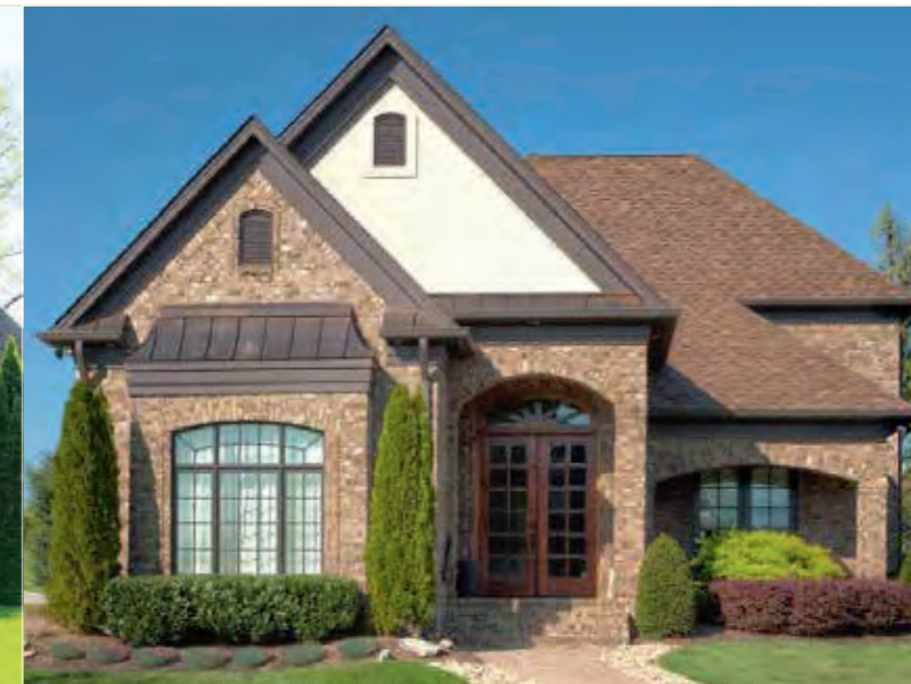
Swing Door Replacement
