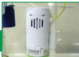
In order to assure proper functioning of the flush valve, the water level in the tank should be over the top of the flush valve. Gravity fed toilets require top water pressure to insure peak performance. **NOTE: Adjust the fill valve to change the water level in the tank if needed.**
