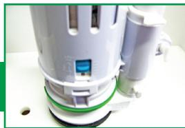
The blue tab on the side of the flush valve can be used to bring more or less water into the flushing system. Pushing the tab down will add more water, while pushing the tab up will reduce the amount of water used.
