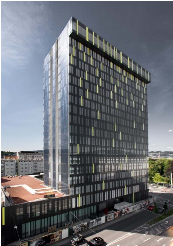
Power Tower, Linz, Austria
