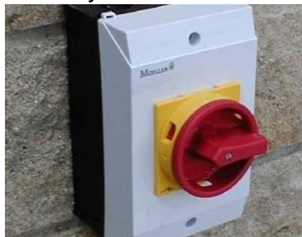
Rotary Isolation Switch
