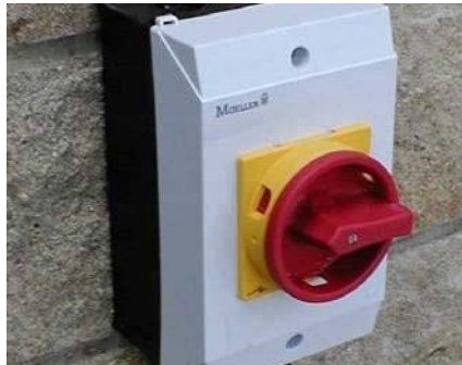
Rotary Isolation Switch
