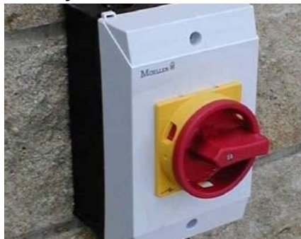
Rotary Isolation Switch
