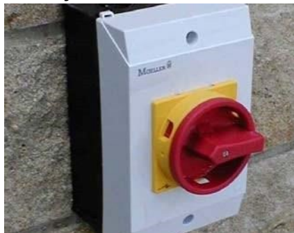
Rotary Isolation Switch
