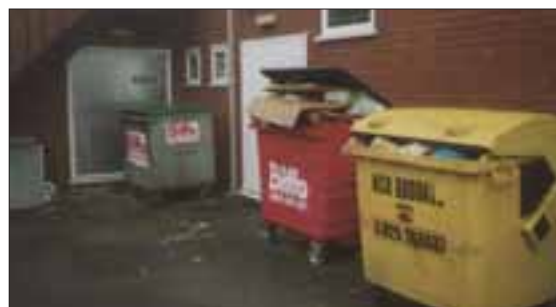
Figure 12: Bins next to a building (courtesy of Cheshire fire and rescue service)
