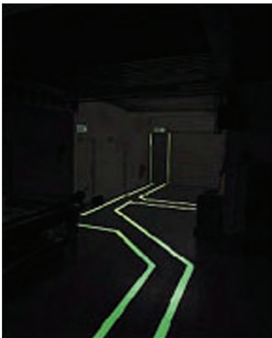
Figure 55: A 'way-guidance' system
