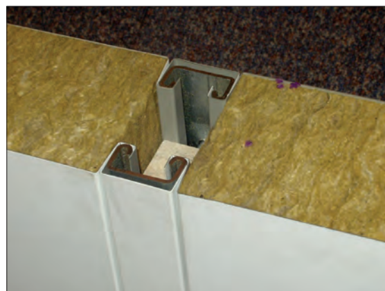
Figure 17: Insulated core panels – internal
