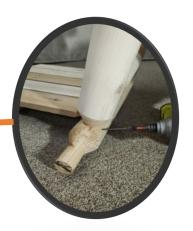
Step 4. Insert the 2 tenons from the Chair Seat (B) into the 2 holes in each Rocker leg (C) and (D)
