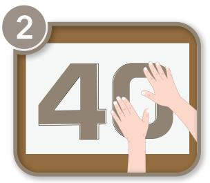
Gently press down on the sign. The studs attached to the back have sharp points to pierce the paper, precisely marking their location.
