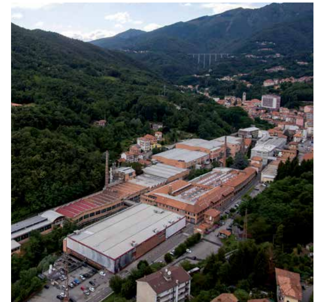
The Vallemosso facility in the province of Biella
