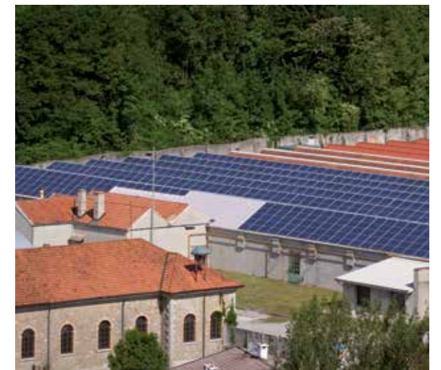
The Tarcento facility "Cascami Seta" in the province of Udine
