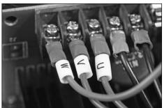
Remove the 4 screws that hold the main circuit board inside the electrical control box and gently pull out the circuit board to gain access to wire terminals. Locate the 5-slot (screw type) terminal post. **N** and **L** are already installed. Install **W**, **V** and **U** cables to their terminals. Note: the cables are marked accordingly.
