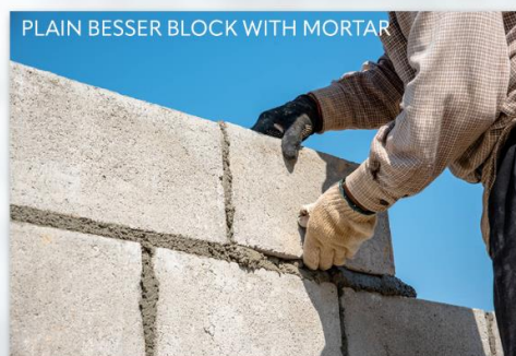
PLAIN BESSER BLOCK WITH MORTAR
