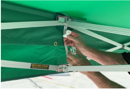
10. Ensure protective flaps are over the truss connectors. Attach them by looping the straps around the truss and engaging the clips, then tighten.
