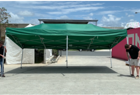
11. Stand on the foot plate and extend front corner legs to desired height.
