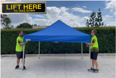
5. Push to release all roof connector pins and refer to the 'LIFT HERE' To Take Down' sticker on the Marquee. CONTINUE TO NEXT PAGE >>
