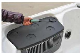
**Step 1.** Remove the two screw cap covers
