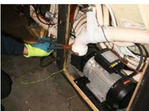
**STEP 9** - Undo pump union joints using an oil filter grip (available at large hardware retailers).
