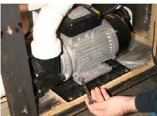
**STEP 8** - Remove all 4 nuts from pump base using a 5/8”(13mm) wrench
