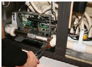
**STEP 8** - Undo left and right side heater unions using large grips
