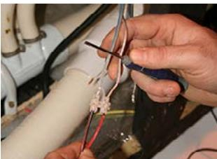
**STEP 9** - Insert wires into 5A connection blocks (Red to Brown and Red/Black to Grey).
