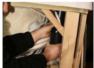
**STEP 4** - Using body of speaker unscrew by turning anti-clockwise (Note: the nut is 'silliconed' in place')
