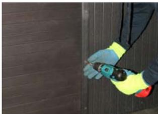
**STEP 1** - Unscrew side panels to access pump on the fascia with air vent and the MP3 Player housing
