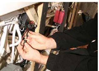
**STEP 4** - Disconnect power supply lead from amplifier by pulling plugs apart.
