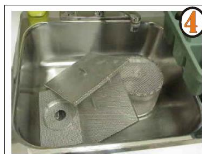
Clean the screens and wash tank of debris. Rinse wash tank. Be careful not to push food debris down the drain.
