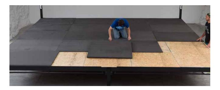
Measure 4" x 4" using square and cut out a corner in the foam pieces around the outer ring posts.
