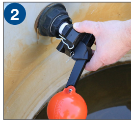
2 Screw in the float valve by hand, valve is suitable for final tightening with a wrench
