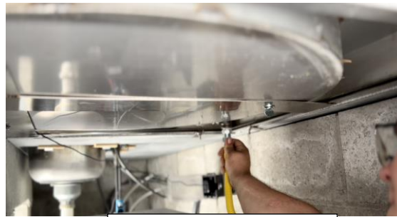
9- Tighten gas line to bottom of hearth
