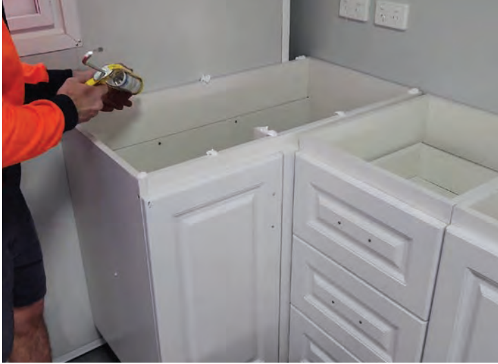
Adhesive for small benchtop piece
