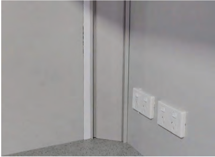
Fitted corner trim piece at 45° angle
