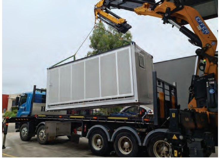
Crane truck shipping for VIOLET unit
