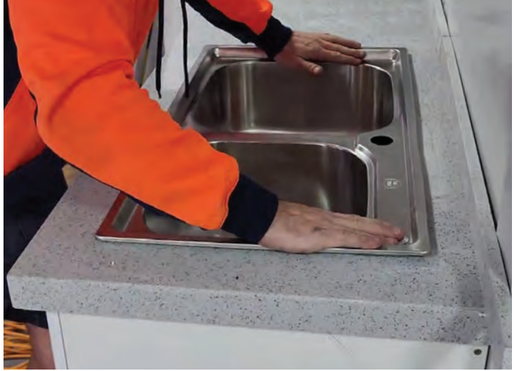
Drop-in sink and apply pressure to bond
