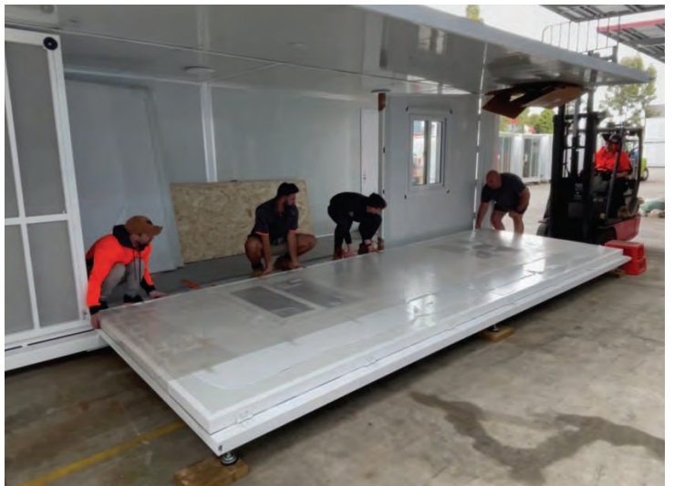
Tape fitted; preparing to raise long wall
