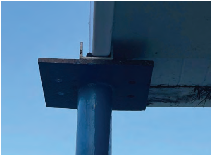
Acrow prop with holder for roof section
