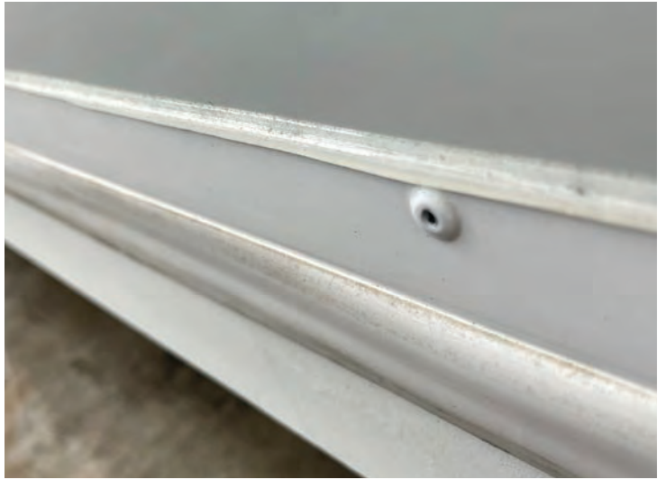
T-mould fitted to the front of the unit; silicon applied above the T-mould
