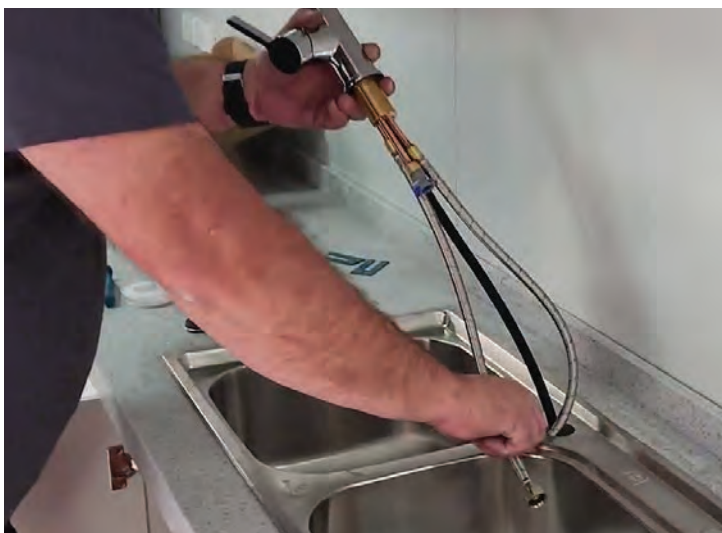
Mixer tap being fitted through sink cutout
