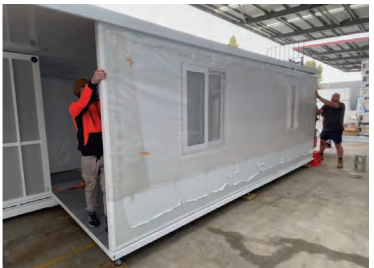
Roof slowly lowered down, support removed
