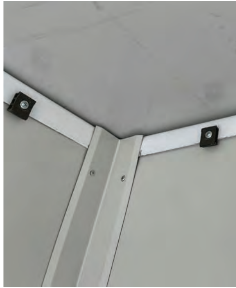
Trim piece locations; Cornice trim wall clips fitted; End cap on trim at door jamb
