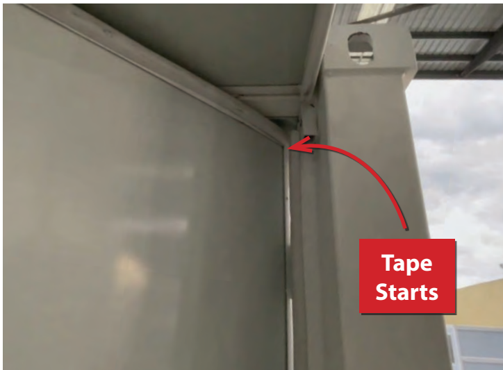
2. Horizontal D-mould fits to outside-facing top edge of short wall, butts up against roof lip
