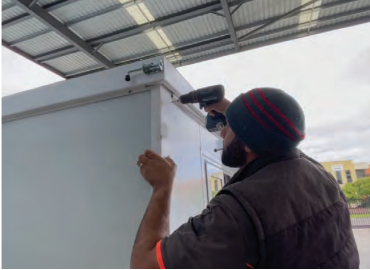
Fastening tek screw at front of unit
