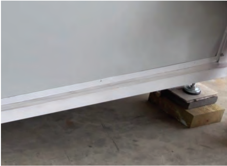
T-mould fitted to the front of the unit; silicon applied above the T-mould
