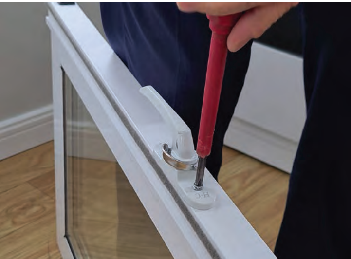
Fitting window latch with screwdriver
