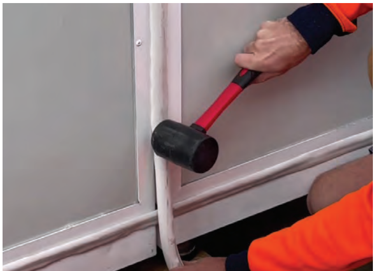
T-mould fitted at long wall join for 40ft unit; T-mould stem cut to fit around other seals
