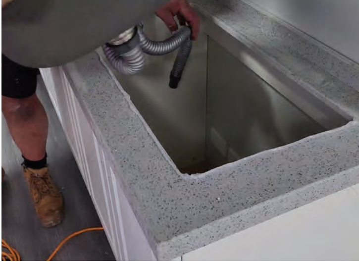
Apply silicon to countertop sink cutout
