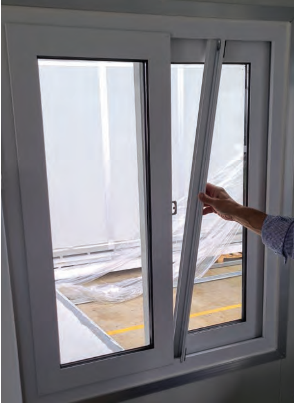
Fitting the window siding to the window
