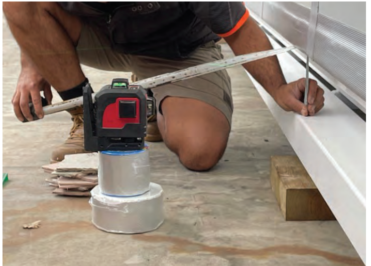
Measuring against laser for unit frame level
