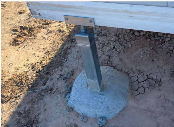
Concrete pad and house stump footings
