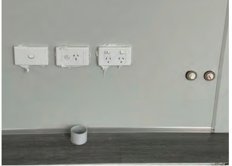
Layout cabinets, take note of inlets/outlets
