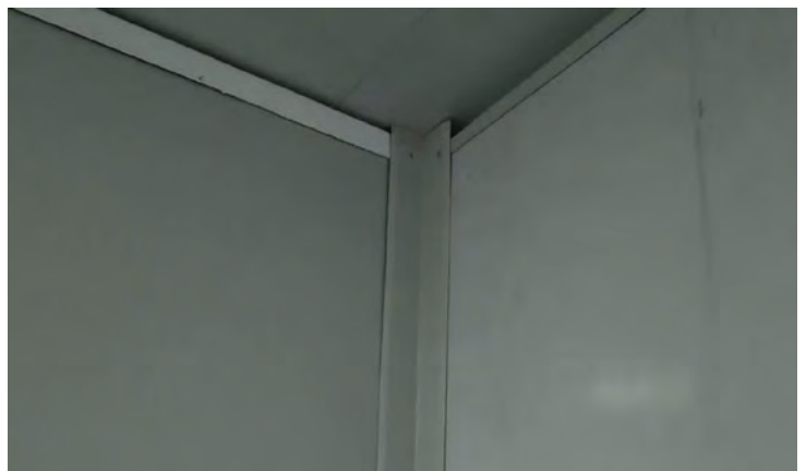
Partition wall L-channel fitted at top
