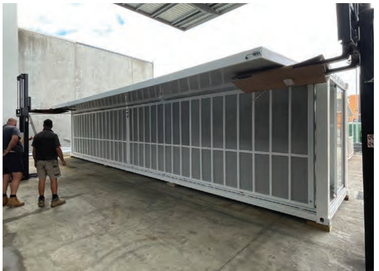
Ceiling raised and supported by forklifts
