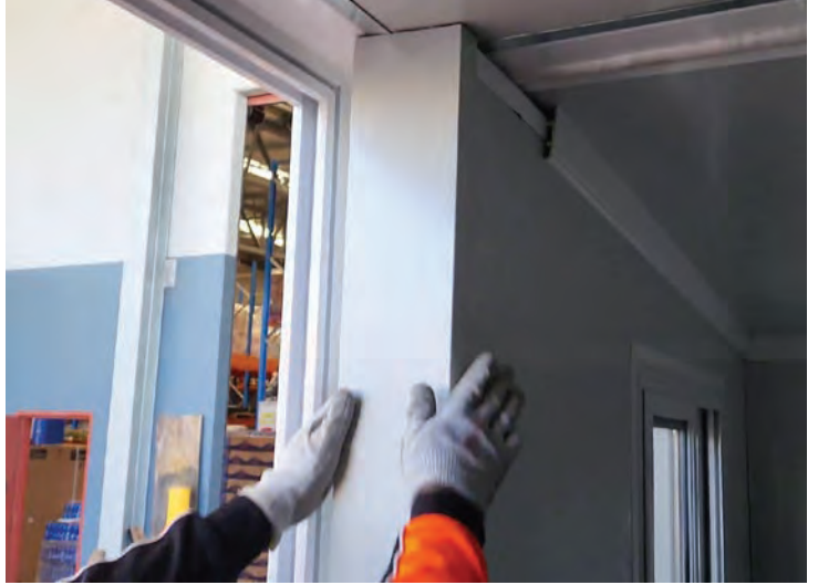
Flashing dry fitted over entry hinge
