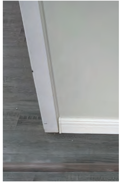
Trim piece locations; Cornice trim wall clips fitted; End cap on trim at door jamb
