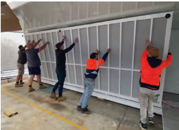
Slowly lowering the floor section
