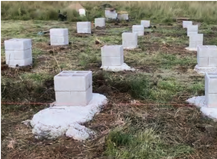
Besser block footings with string lines
