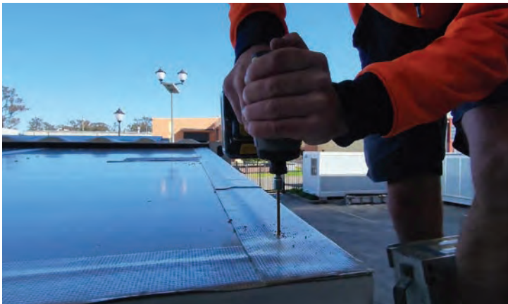
Partition wall L-channel fitted at base
