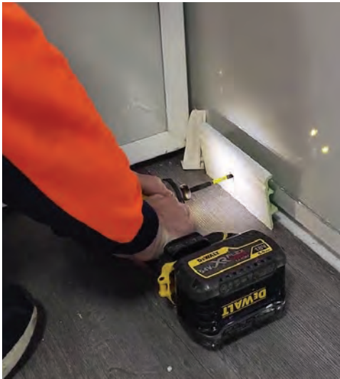
Trim piece locations; Cornice trim wall clips fitted; End cap on trim at door jamb
