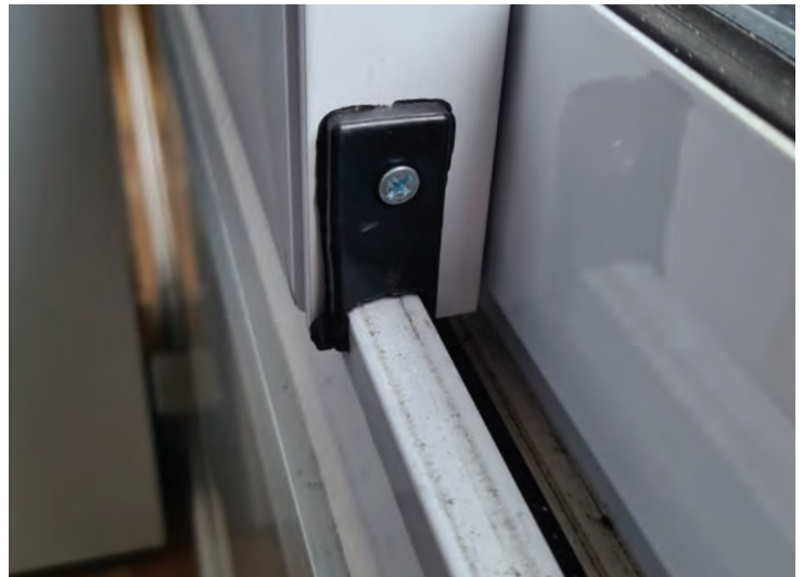
Gap cut in siding plastics to suit rails
