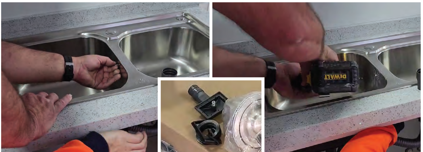
Fastening overflow connector with included screw through the overflow grill on the sink
