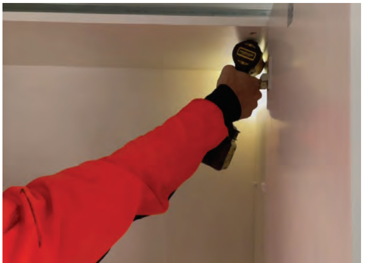
Fastening cabinet assembly to the wall
