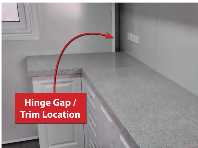
Corner trim location and cut-to-size corner trim being inserted into place
