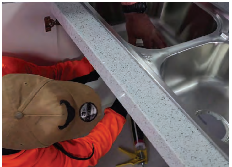
Drain fitted over silicon bead, pressure applied, plastic nut screwed on underneath
