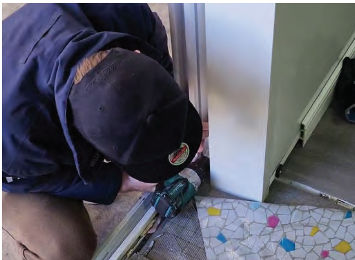
Pilot hole, bottom of doorway side
