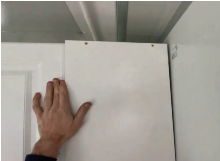
Ensure a good connection to hooks
