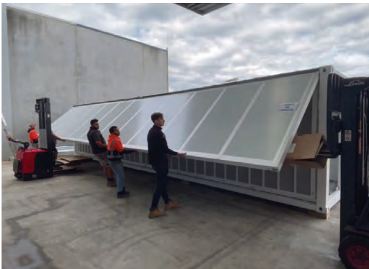
Raising 40ft VIOLET unit roof with forklifts
