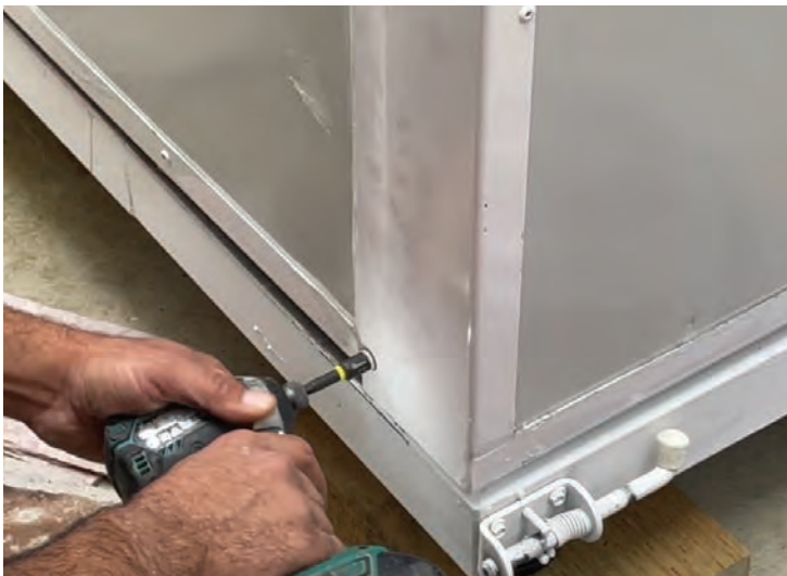
Fitted through long wall lip into short wall
