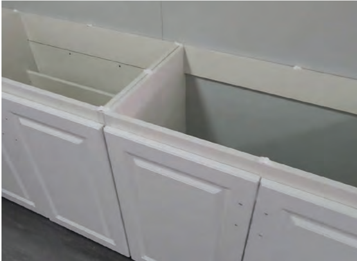
Adhesive for large benchtop piece
