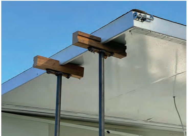
Acrow props with holder for roof section
