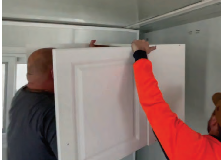
Mounting first cabinet to wall hooks
