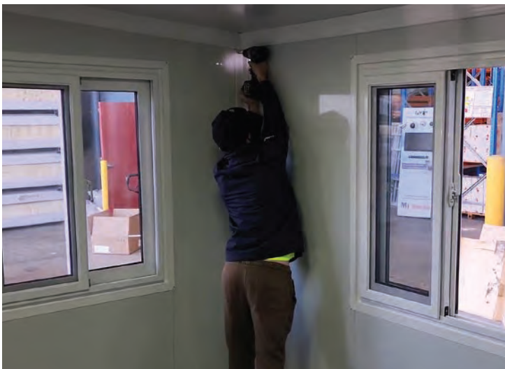
Drilling pilot hole for rivets to secure walls
