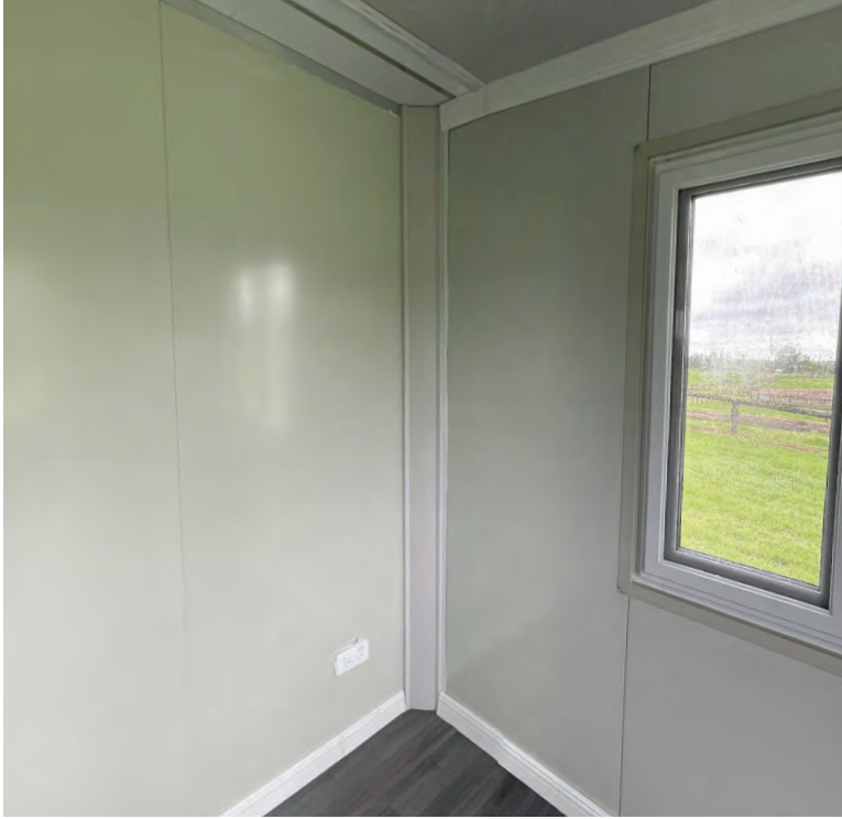
Corner trim pieces fitted to cover hinges in bedrooms (shown with skirting trim fitted)
