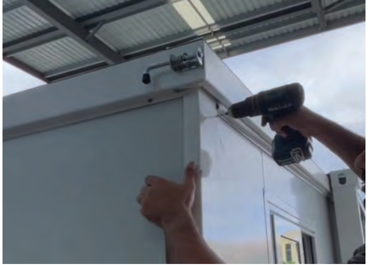
Fitted through long wall lip into short wall
