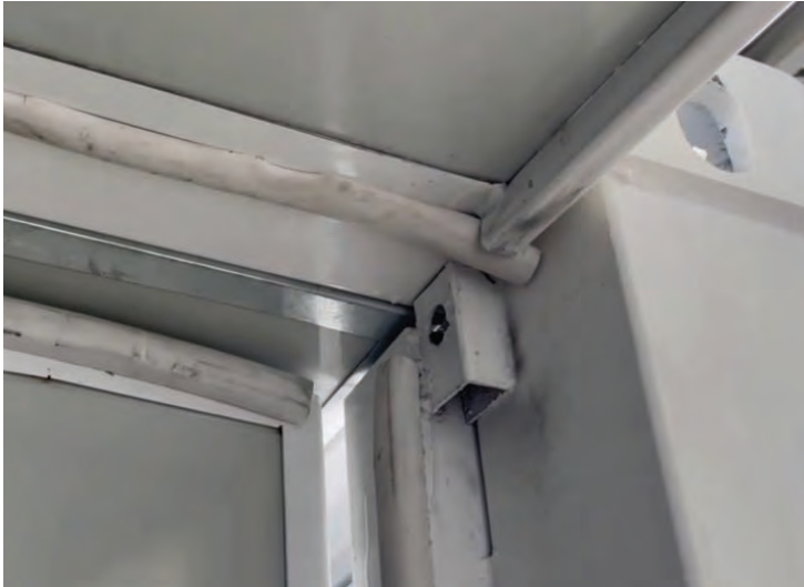
Ceiling T-mould fitted to cover the gap
