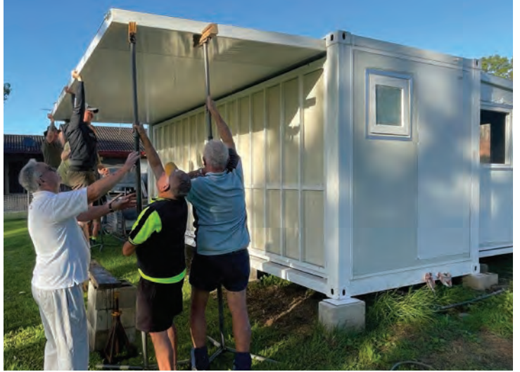
Raising roof and placing props beneath
