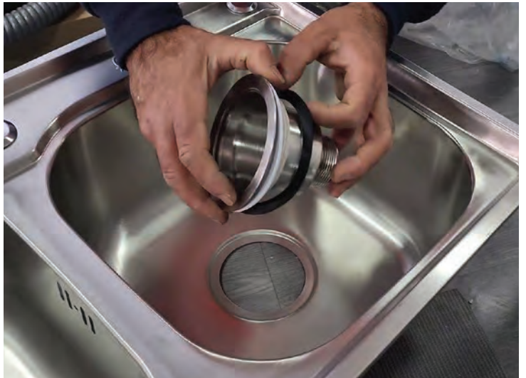
Take rubber washer from plug, fit to underside and screw on connector to secure
