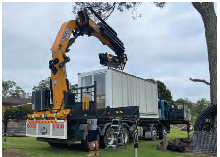
Crane truck preparing to lift-off unit
