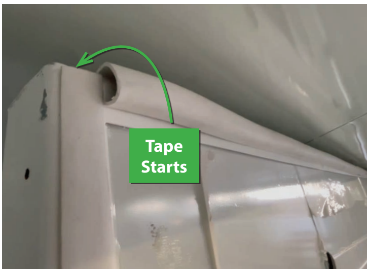
3. Vertical flat tape fits to outside-facing outer edge of short wall, butts up against long wall
