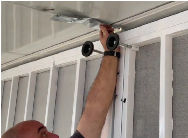
Removing exterior bracket (40ft)
