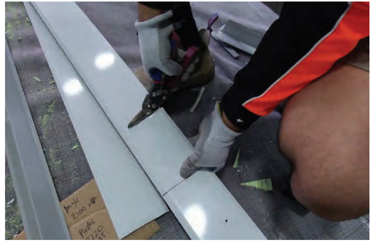
30ft/40ft unit interior flashing measured and cut to size using tin snips
