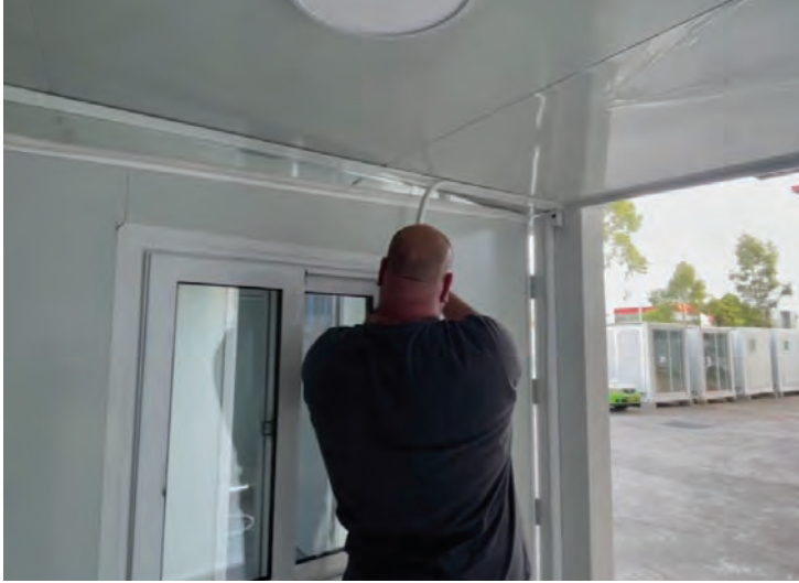
Ceiling gap to be sealed by T-mould
