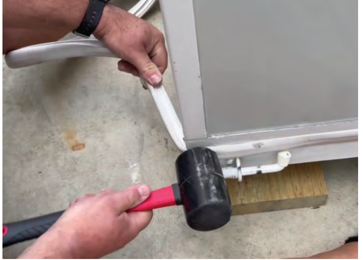
To fit around corners, cut the T-mould stem at a 45° angle and fit with rubber mallet
