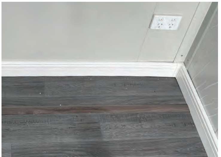
Floor trim fitted after fitting skirting trim
