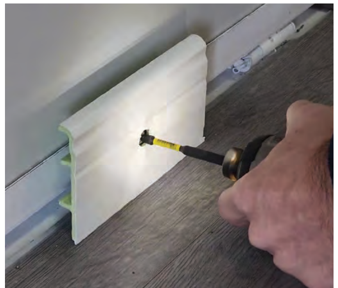
Using trim piece with hole as a drill jig
