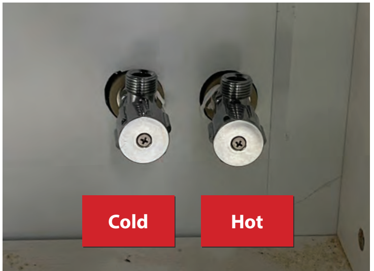
Remove stops and connect taps for hot/cold
