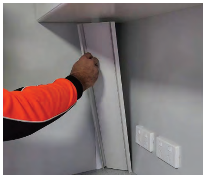
Corner trim location and cut-to-size corner trim being inserted into place
