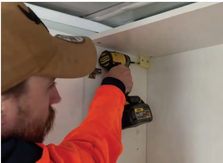
Pre-fitted guide block to assist in fastening
