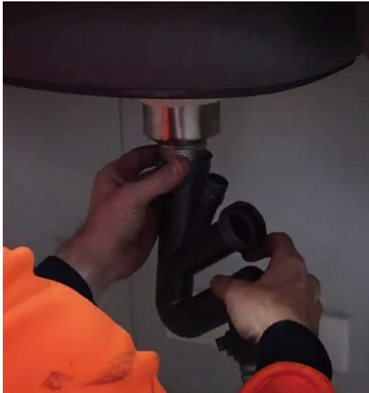
Fitting the drain collector, overflow flex-hose, small basin flex-hose and greywater flex-hose
