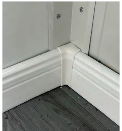
Trim connector pieces clip in between straight pieces and in corners
