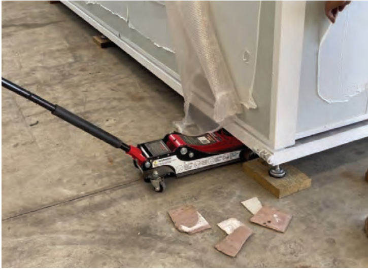
Trolley jack & shims to adjust corner height
