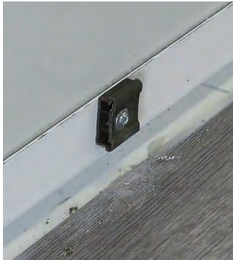
Fitting the trim clips to the wall using the jig
