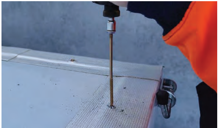
Partition wall L-channel fitted at top
