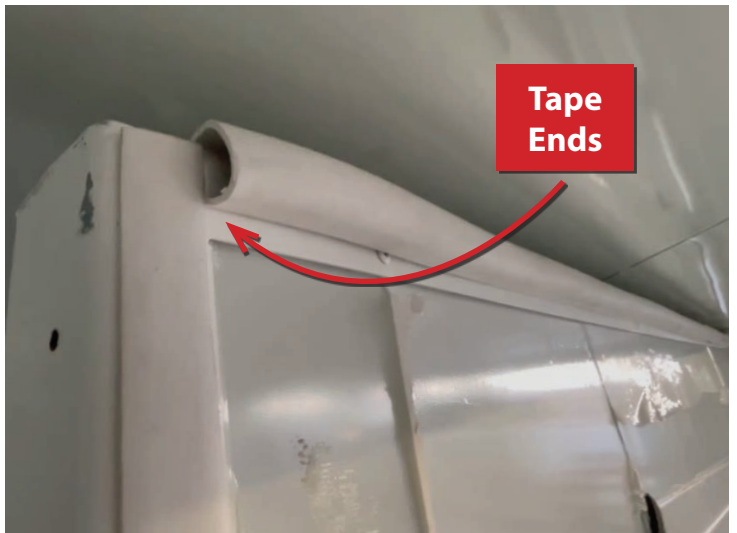
2. Horizontal D-mould fits to outside-facing top edge of short wall, butts up against roof lip
