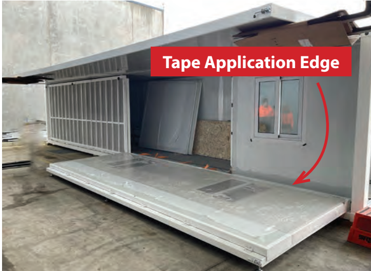
Wall/floor section lowered ready for tape
