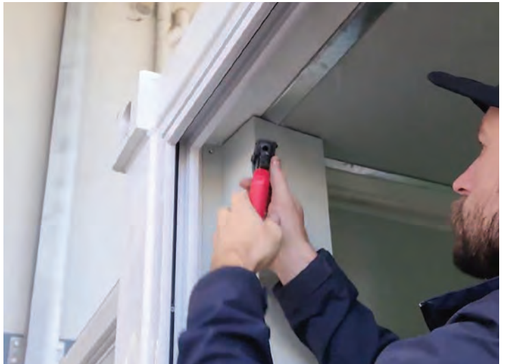
Rivet, top of doorway side
