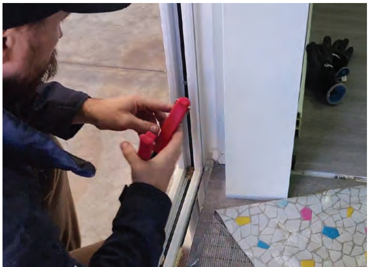
Rivet, bottom of doorway side
