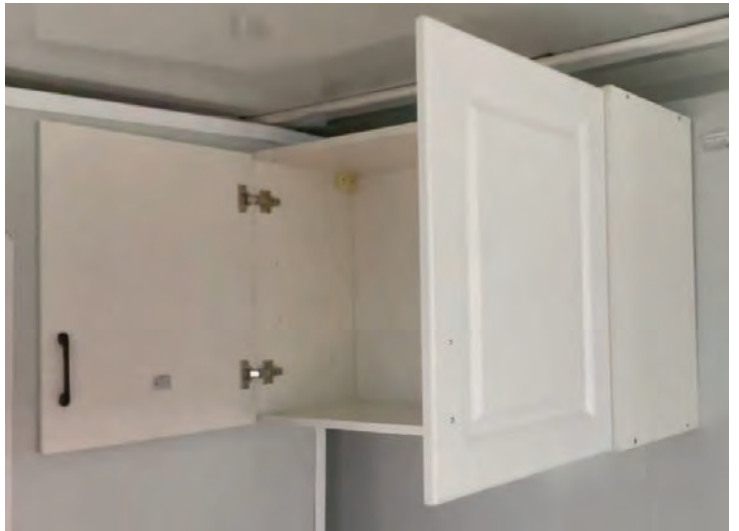
First cabinet mounted on wall hooks
