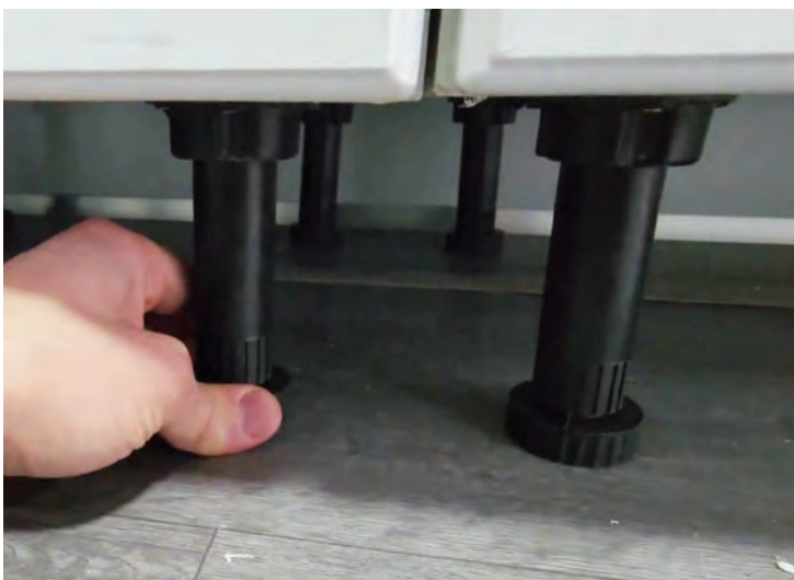
Make level with feet screw adjustment
