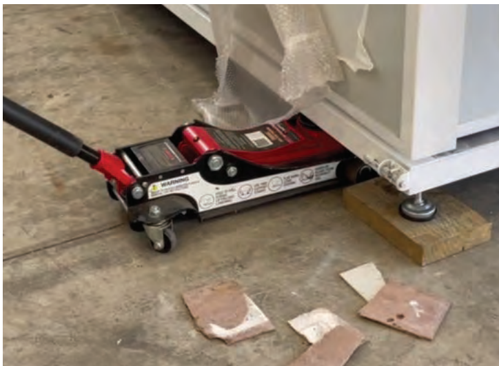
Trolley jack to assist in raising unit edge
