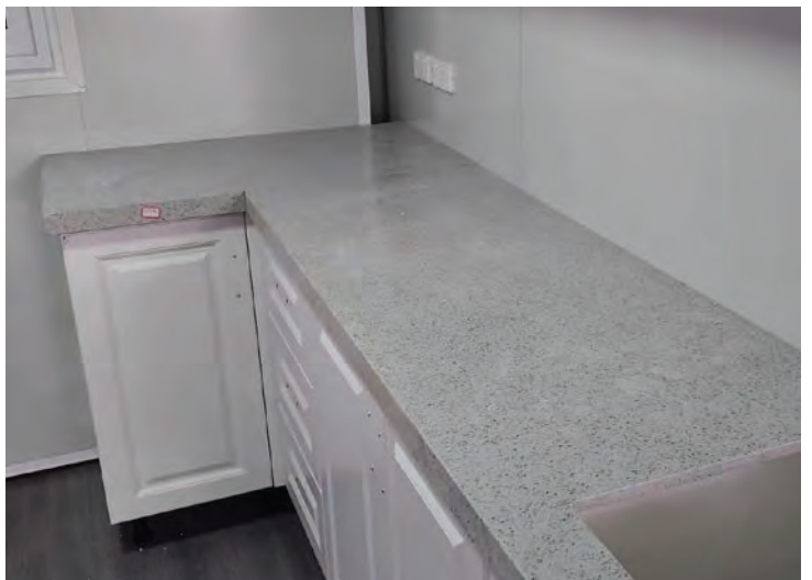
Benchtop fitted, excess adhesive cleaned
