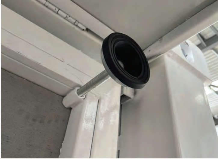
Fitting screw in feet to floor before lowering
