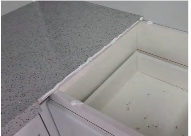
Benchtop join rough edge with adhesive
