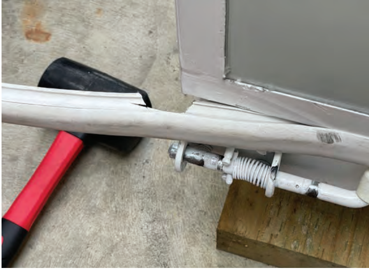
To fit around corners, cut the T-mould stem at a 45° angle and fit with rubber mallet
