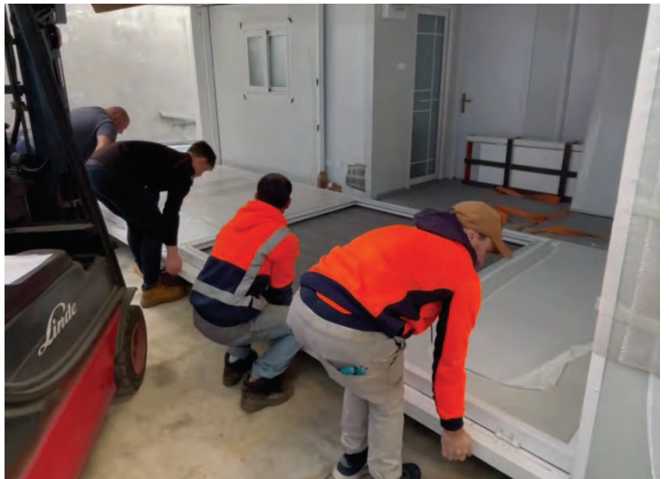
Supports out of way of workpath as lowered
