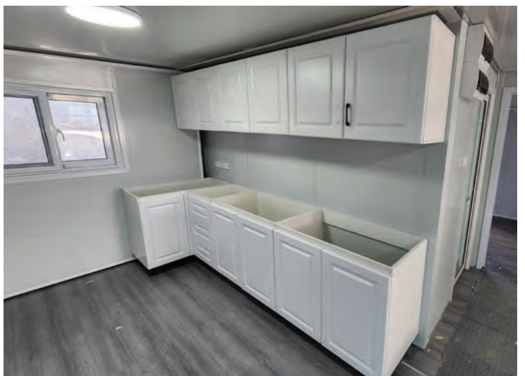
Fitted kitchen cabinets for 40ft unit
