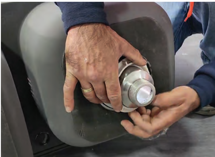
Drain fitted over silicon bead, pressure applied, plastic nut screwed on underneath
