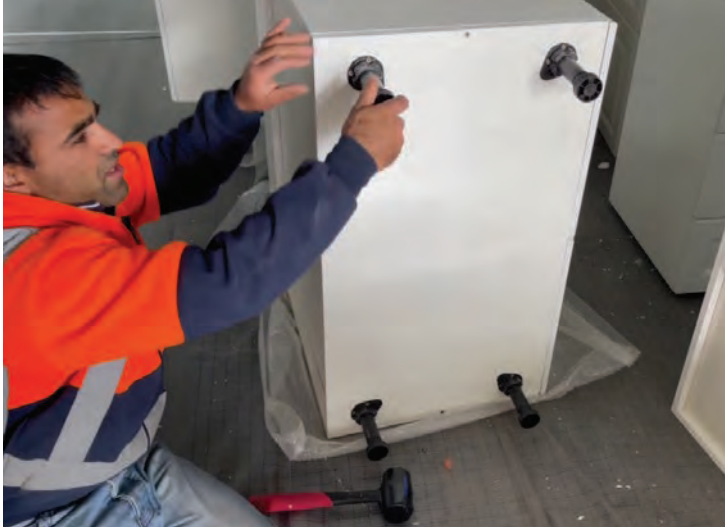
Push in cabinet feet and add screw base
