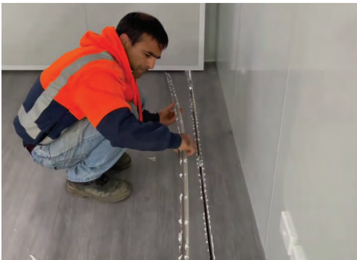
Preparing to stick down the floor trim
