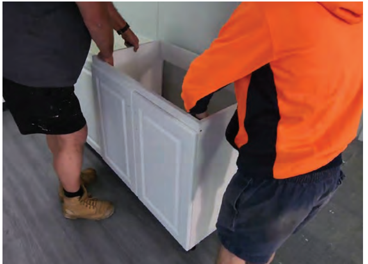
Move each cabinet into place, butting cabinets up against one another
