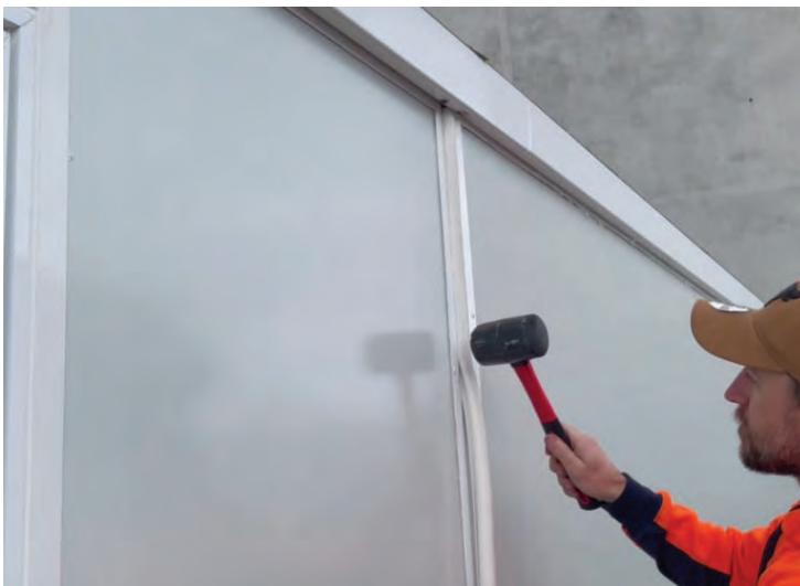
T-mould fitted at long wall join for 40ft unit; T-mould stem cut to fit around other seals
