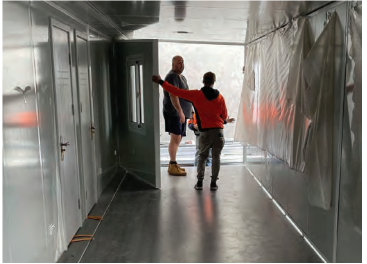
For safety, swing out walls from the interior
