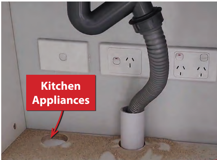
Holes cut for greywater drain with extension
