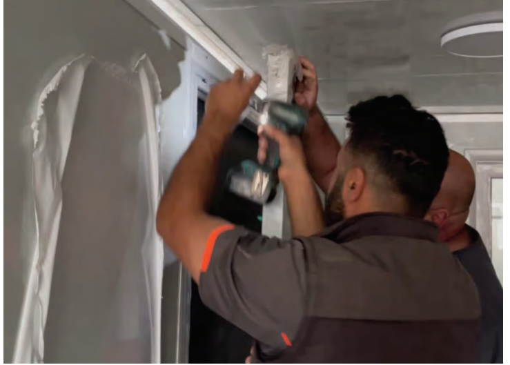
Removing interior brackets (20ft/40ft)
