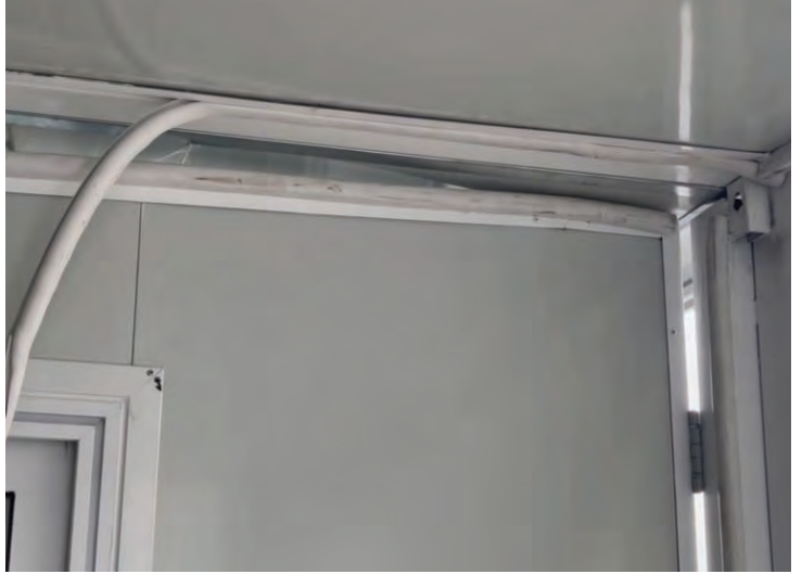
Cut T-mould stem to fit over hinges
