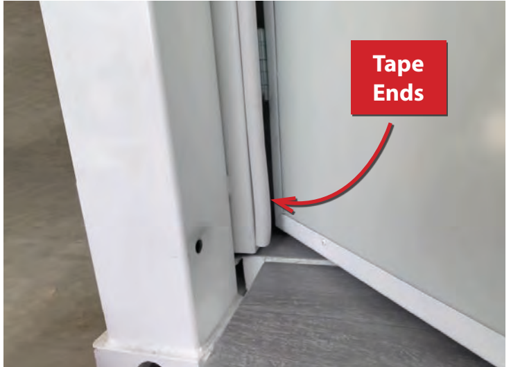
1. Vertical D-mould fits to the inside centre frame, butts up against closing short wall
