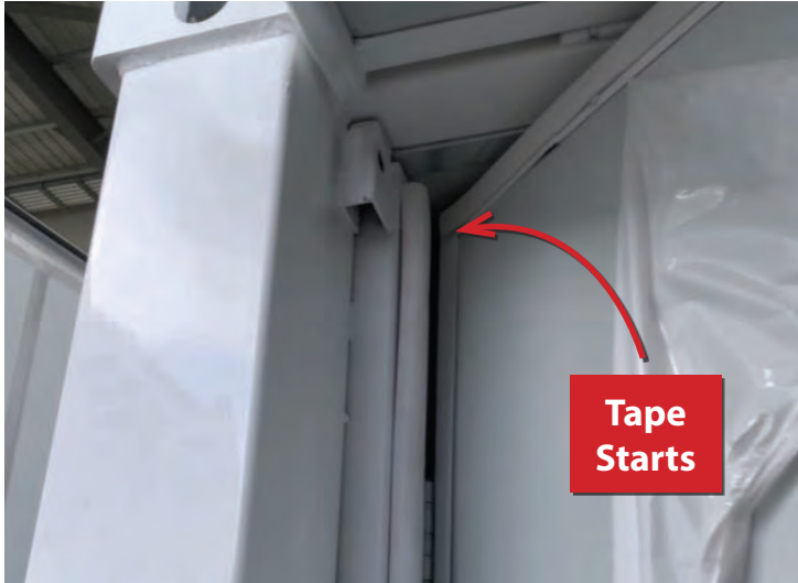
1. Vertical D-mould fits to the inside centre frame, butts up against closing short wall
