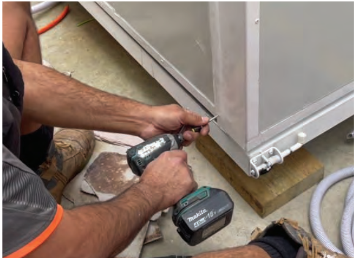
Fastening tek screw at rear of unit
