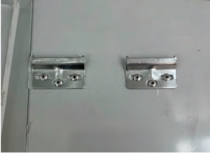
Pre-fitted hooks for mounting wall cabinets
