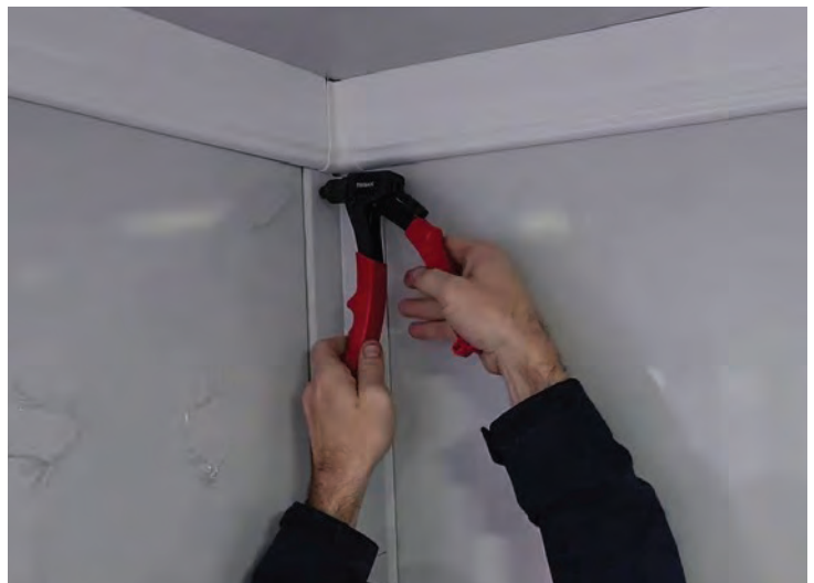
Fastening walls together with rivets
