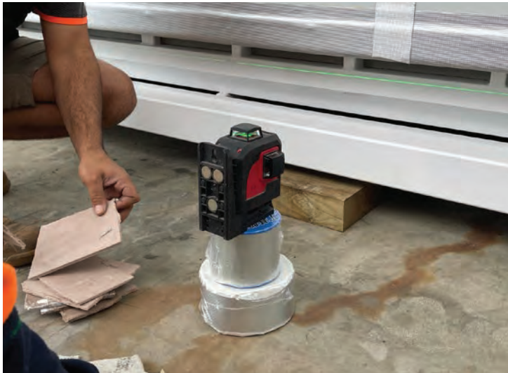
Plane laser level and fibreboard shims
