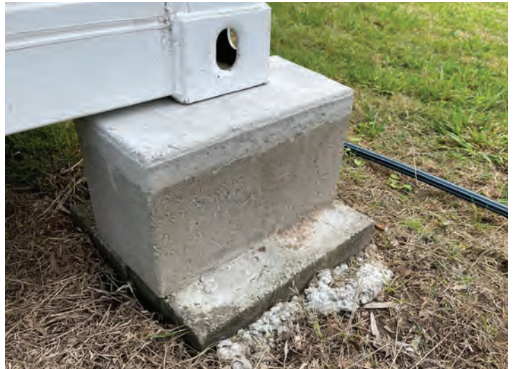
Dug-in besser blocks and concrete footing
