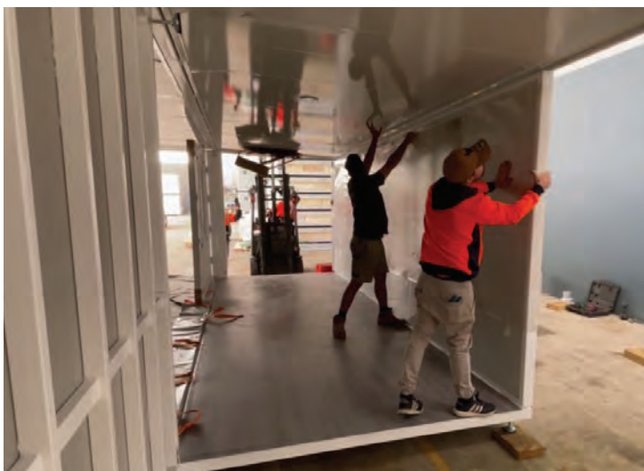
Guide wall from both interior & exterior
