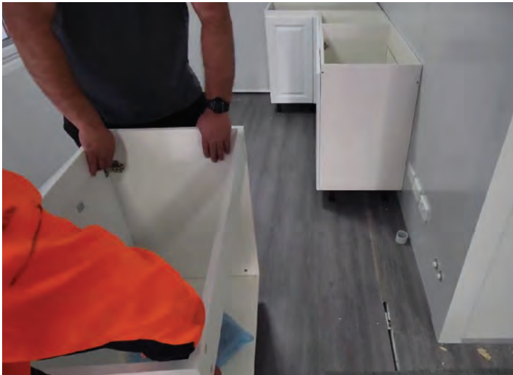
Move each cabinet into place, butting cabinets up against one another
