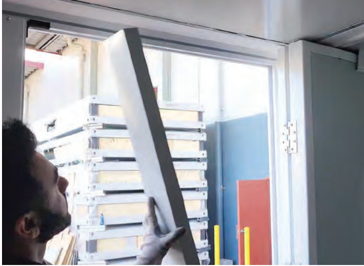
Fitting flashing over entry hinge
